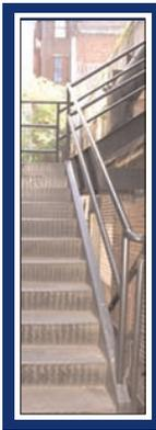
Galvalox is organic and contains over 90% zinc in the dried film which protects the steel substrate by acting as a sacrificial coating. Galvalox prevents rust creepage and undermining.
